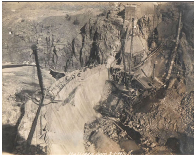
Arch halfway built - looking east
