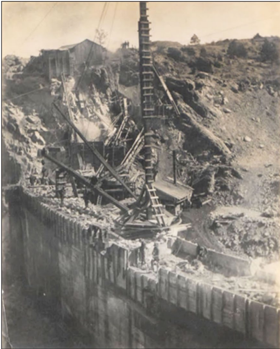
Building up the base
